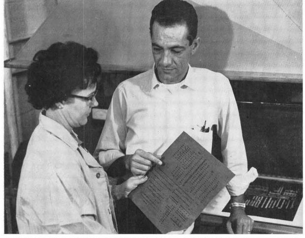
NEW PHOTOSENSITIZING technique for numbering circuit boards, discussed here by Don Tassano, right, and Jessie Berry, both of 8223-3, requires only one man-hour for entire process. Negative used to expose numbers on plate is shown in this photo on the light table behind Don.
